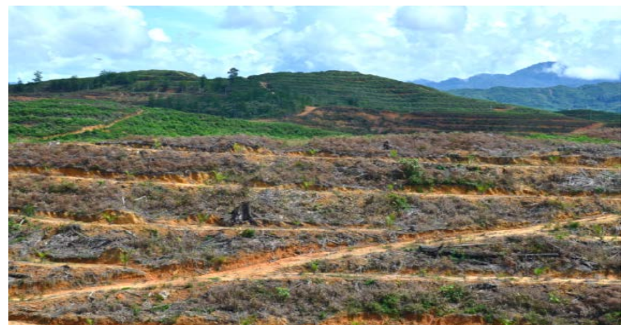
Clearing and terracing of plantation land
